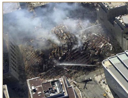
Total dismemberment of steel structure – fell like a house of cards
